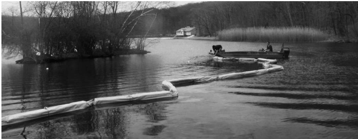
Figure 2. Installation of a limnobarrier around an island in Crystal Lake, Connecticut.
